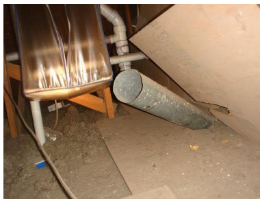
BATHROOM VENT PIPE
