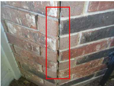
MORTAR MISSING
